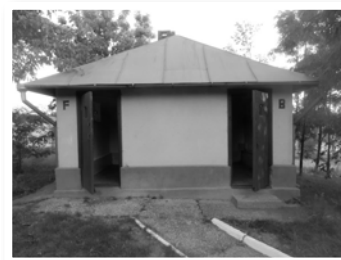
The finished toilet block at Slovenca
