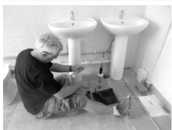
Installing basins at Mindresti Noi
